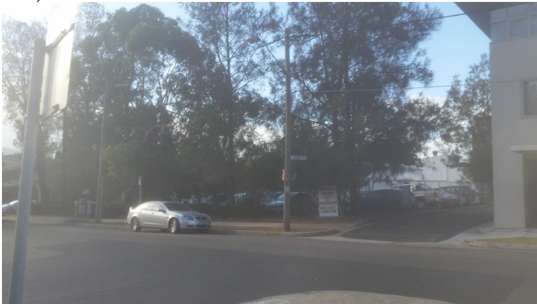
Fig.13 Photograph of hardstand car park at 2 Hogben Street and 127 Princes Highway, Kogarah
