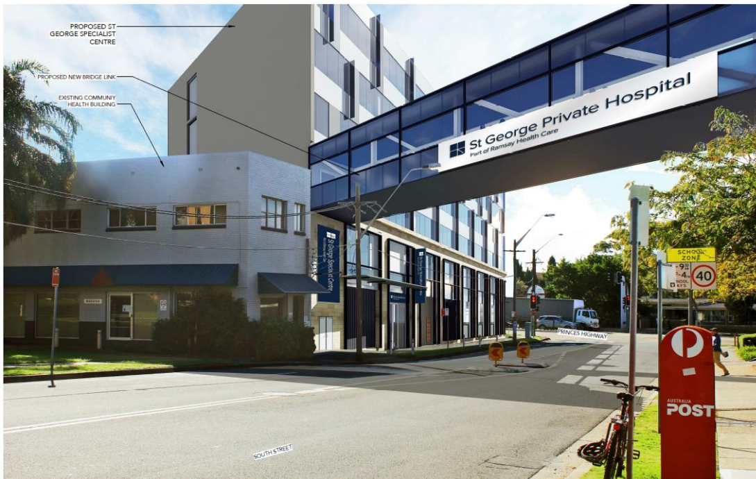
Fig.7 Montage of proposed pedestrian bridge linking 131 Princes Highway to 1A South Street which is elevated above South Street (Source: Architectural plans prepared by Team 2 Architects, 2017)
