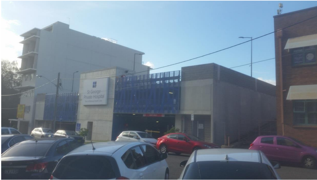
Fig. 14 Photograph of multi-storey car park at 6,6A and 12 Hogben Street, Kogarah
