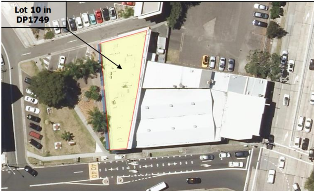
Fig 18. Aerial extract of 2 South Street, Kogarah which adjoins 131 Princes Highway along the western rear boundary.
